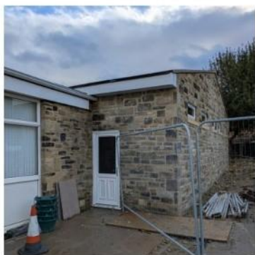
New entrance into enlarged stores from Sun Terrace
