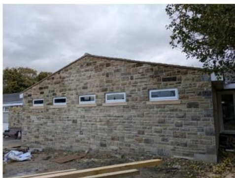
Scaffolding gone and now it can be seen how well the new stone gable matches the original
