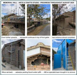
Aided by continued good weather, progress was generally maintained throughout August to the point where all inner and outer leafs of brickwork and stonework are virtually completed. The AIB asbestos has been safely and professionally removed enabling work to start on the roof timbers. It is anticipated that the roof will be sheeted over during the second week of September with windows and doors following soon after.
