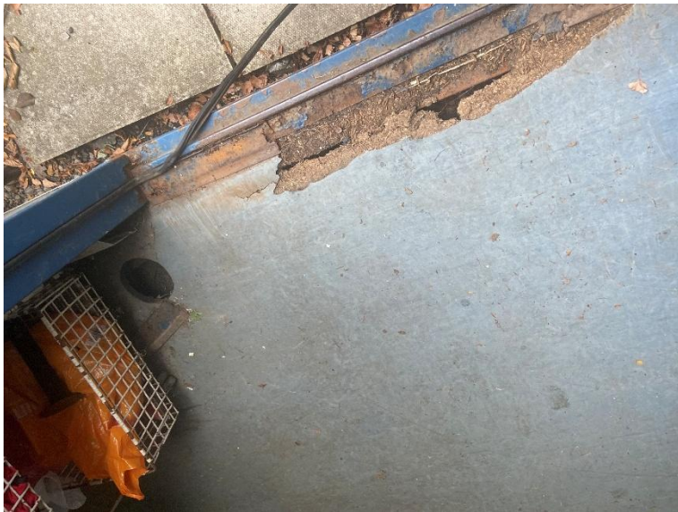
Fig 1 – Floor immediately behind external door to left hand cabin
